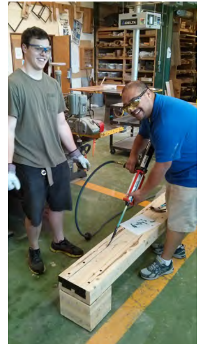
Building the Mockup Bench Photo: A. Schreyer
